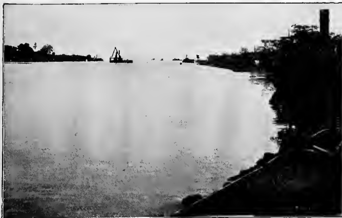
PART OF THE COMPLETED CANAL
